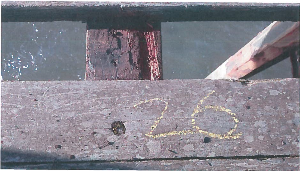
Photo 3 Joist 26 in fair condition. Stress estimated = 0.543
